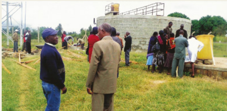
Members of the RuWaSCo outside their offices, and the water treatment unit built through IFAD
